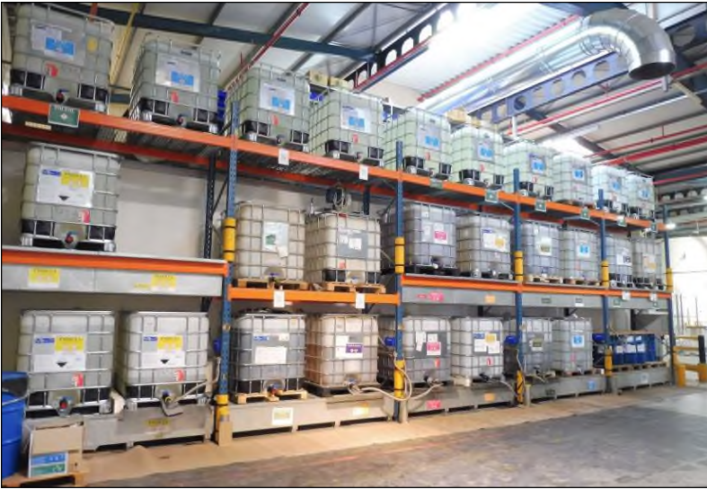
Stockage IBC Hall B
